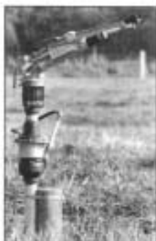
Valve on riser supported by buried post for low cost, effective installation.
