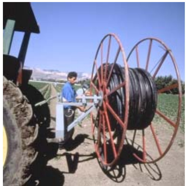
Polyethylene pipe can be installed or retrieved from the field with the aid of a tractor driven reel as shown above.
